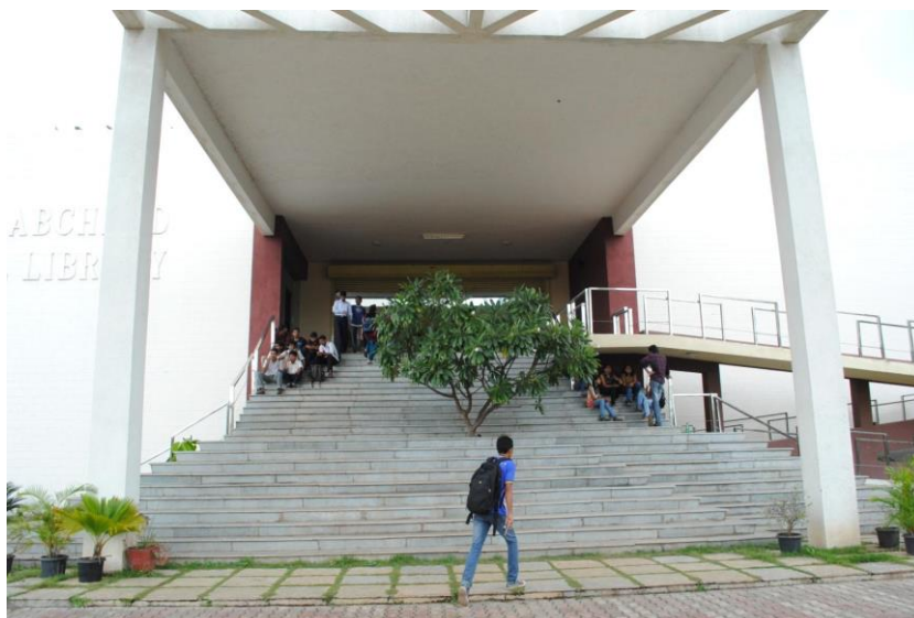
Ramp facility at the right side of the Central Ajit Gulabchand Library
