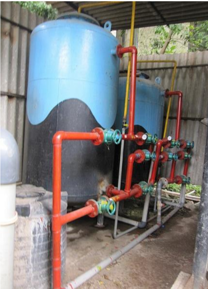
Water Filtration Plant of 50000 liters capacity and Distribution System Power Substation with 325 KVA sanctioned Capacity and Generator set of 125 kVA capacity along with PLC and SCADA system caters to the electricity needs during load shedding.
